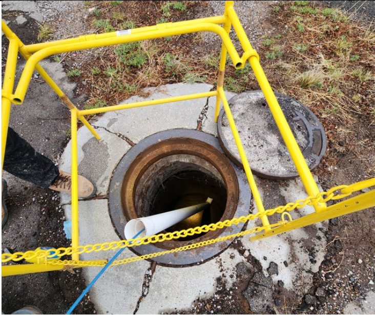
Photo 9: (05/07/2025) Push camera deployed in manhole E-11.
