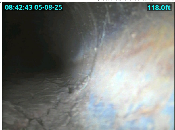
(FC) Fracture circumferential from ... to ... survey00000108/2025_05_08-08_42_43_509.jpg
