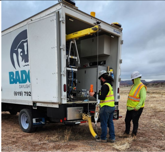
Photo 1: (05/06/2025) Badger crew sets up 8" crawler camera on manhole H-1.
