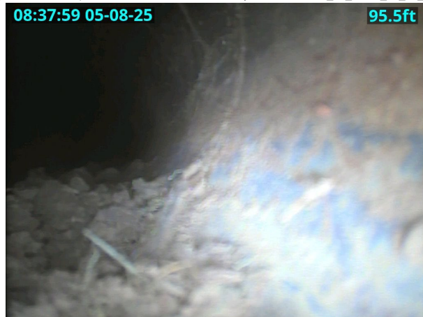
(FC) Fracture circumferential from ... to ... survey00000108/2025_05_08-08_39_15_209.jpg
