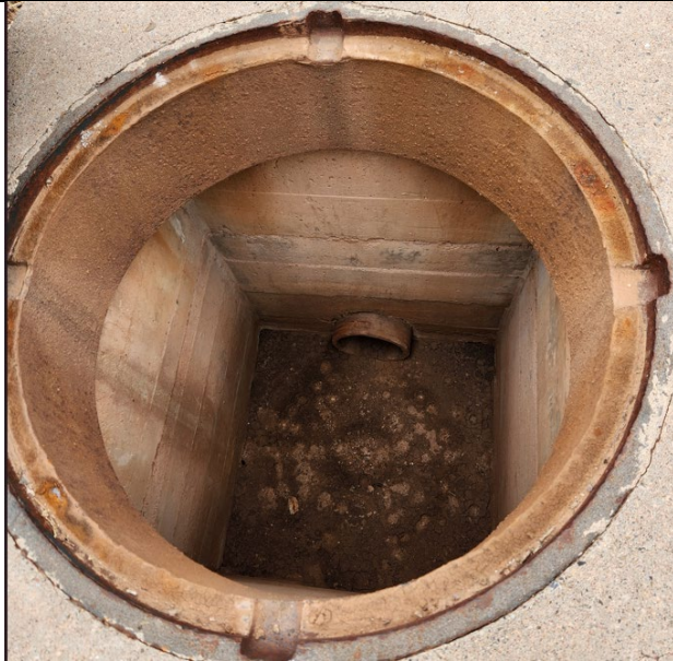
Photo 5: (05/06/2025) Manhole F-14. Access to sewer line unimpeded.
