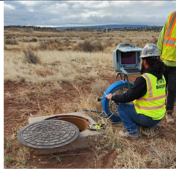
Photo 2: (05/06/2025) Badger crew sets up push cable camera on manhole F-14.
