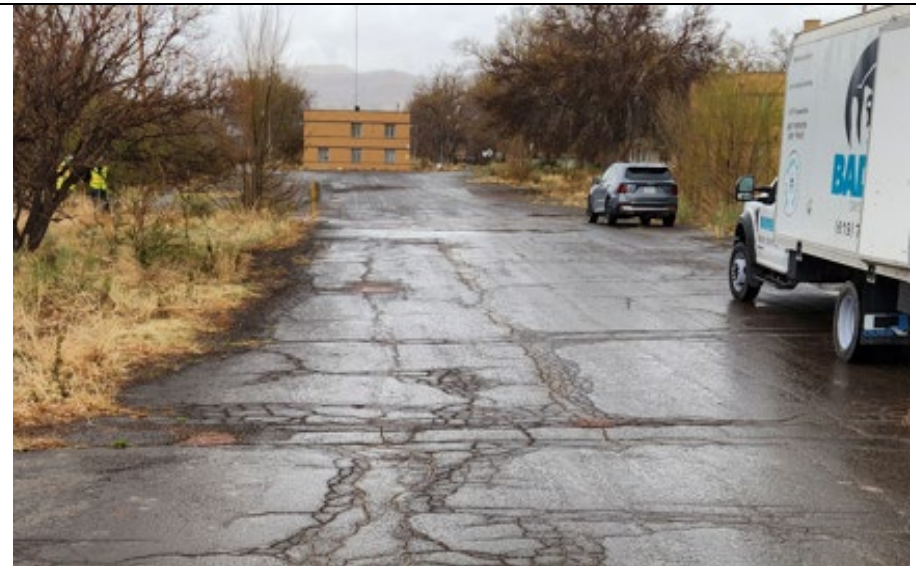
Photo 8: (05/07/2025) Suspected location of covered manholes E-3 and E-4.
