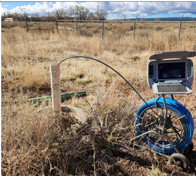
Photo 13: (05/08/2025) Push camera deployed in manhole E-16.
