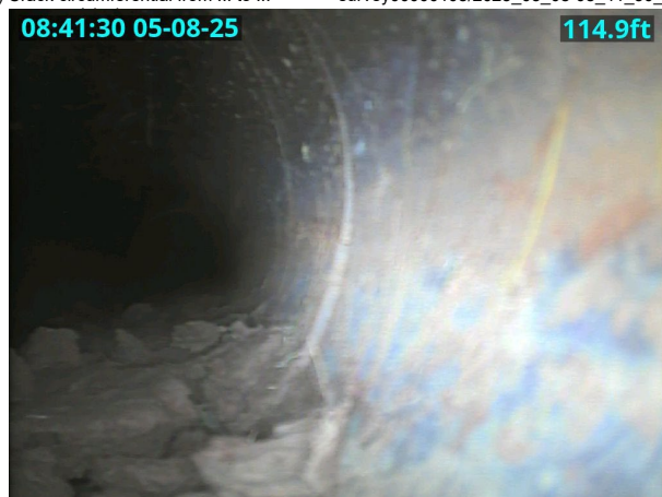
(CC) Crack circumferential from ... to ... survey00000108/2025_05_08-08_43_33_624.jpg
