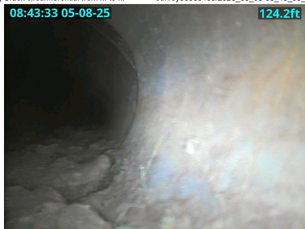
(CC) Crack circumferential from ... to ... survey00000108/2025_05_08-08_43_33_624.jpg
