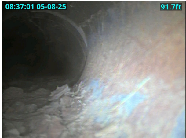
(CL) Crack longitudinal at ... o'clock survey00000108/2025_05_08-08_38_35_330.jpg
