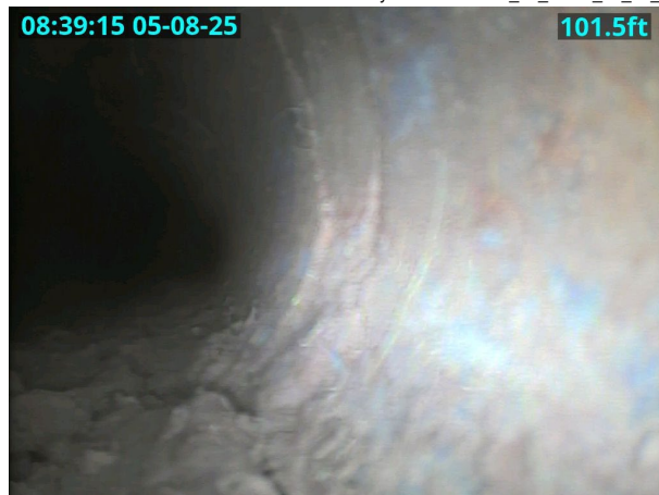
(CC) Crack circumferential from ... to ... survey00000108/2025_05_08-08_41_30_596.jpg
